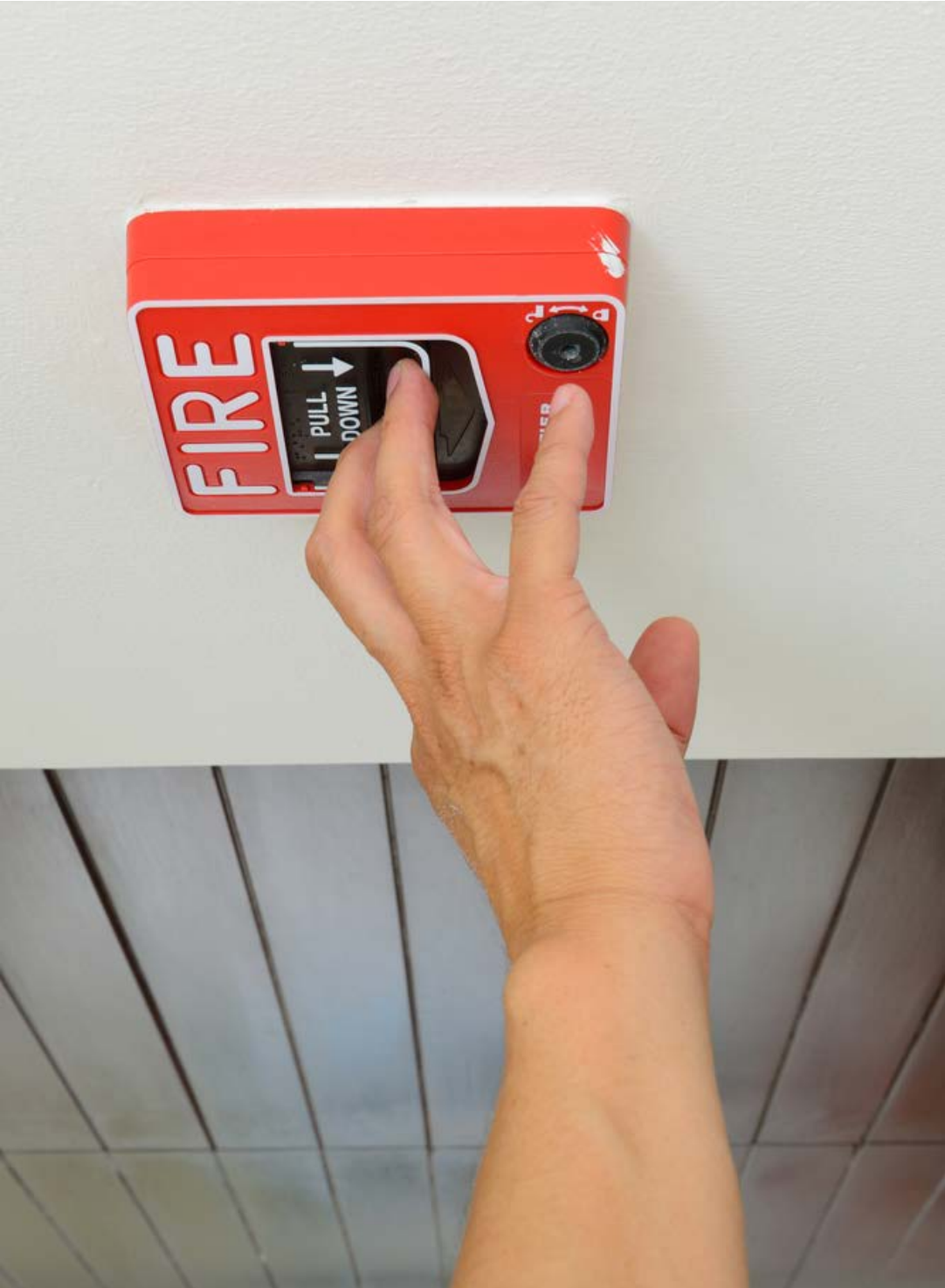
Pull the fire alarm
