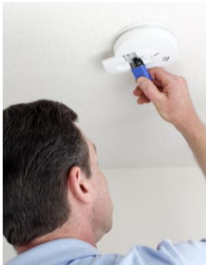
Make sure the batteries are charged
